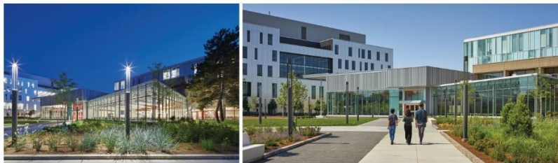
Görsel35. TomArban, Seneca College Newnham Campus Food Hall, 2021, yemekhane cephe görünüşü, Taylor Smyth Architects, Kanada.
